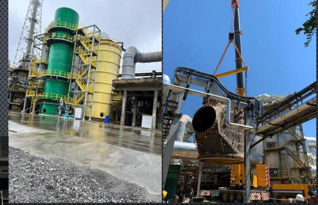
Construction of two additional washing towers to a Sulfuric Acid production facility.
